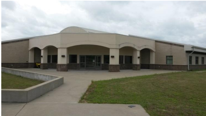
Waynesburg Readiness Center 500 Evergreen Drive Waynesburg, PA 15370
