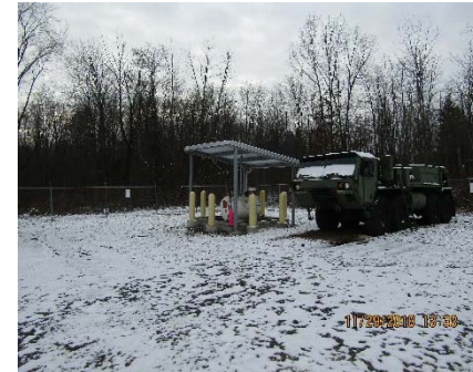
Fuel Point in Gravel MEP Enclosure
