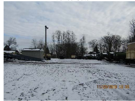
Enclosed Gravel MEP Adjacent/South of Paved MEP
