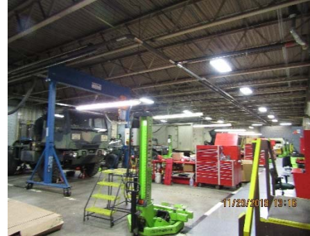
Maintenance Bays – View 2
