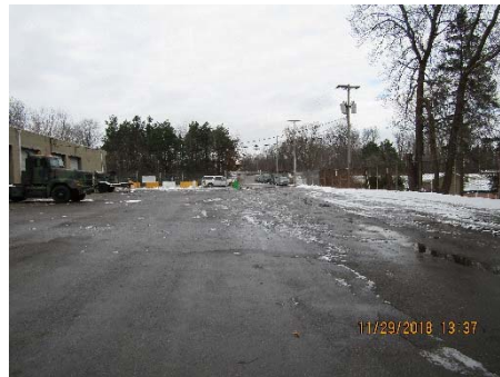
Apron & Roadway Looking North Toward Entrance Gate
