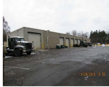
Overhead Entrance to Maintenance Bays
