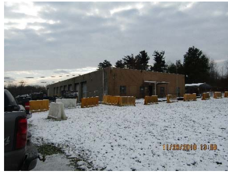
Front Entrance to AMSA 110 Facility
