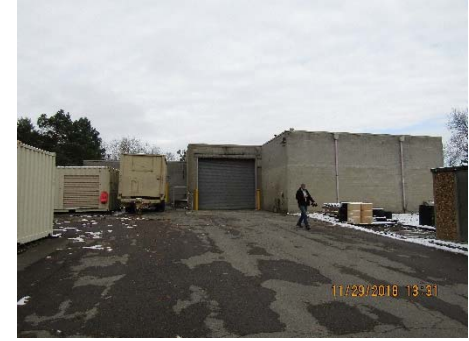
Rear OH Entrance to Maintenance Bays
