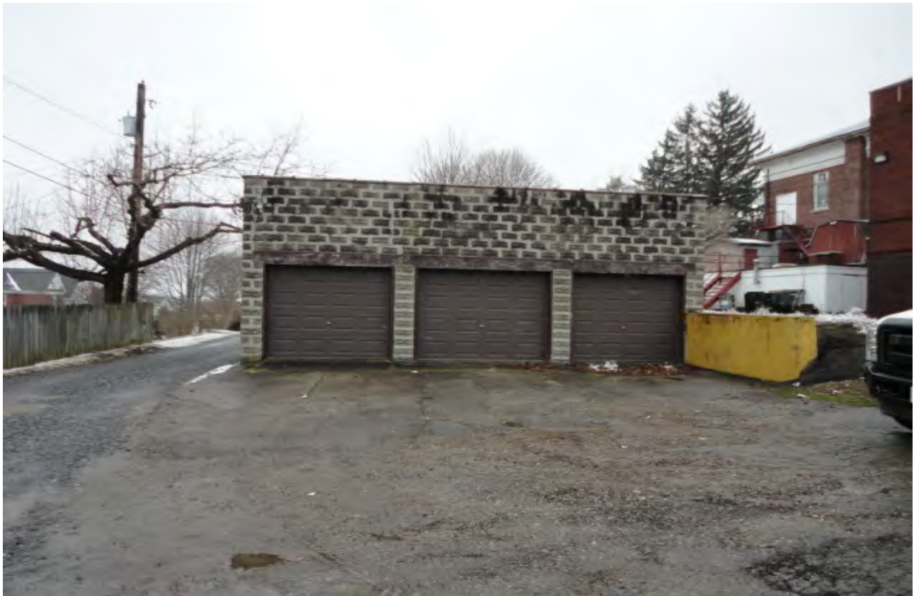
Photograph 4: View to the west of the garage building located south of the RC.
