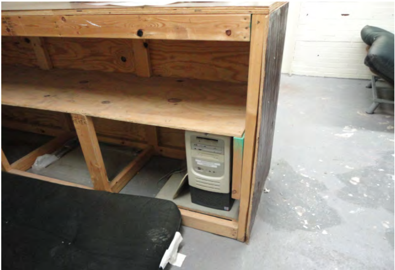
Photograph 10: View of a computer left in the RC basement.
