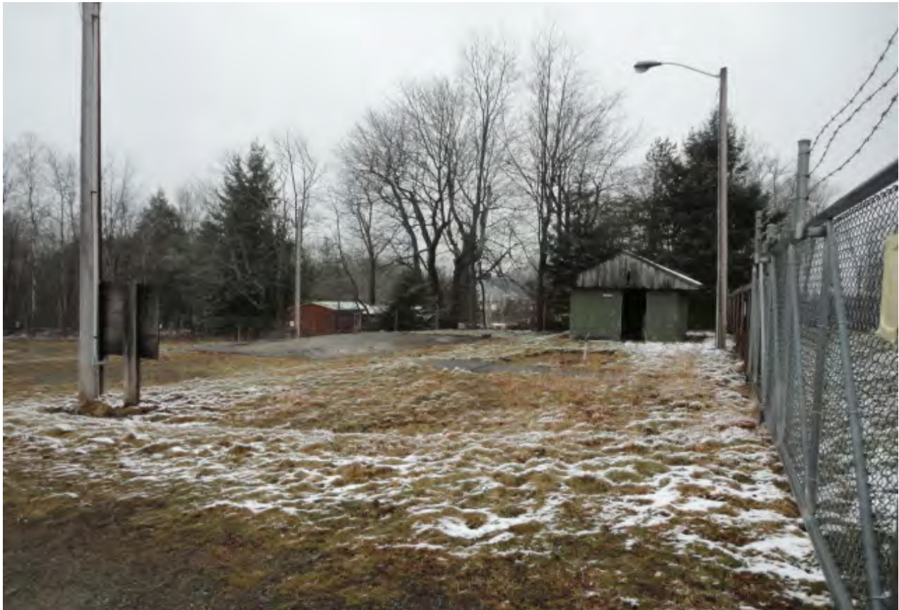
Photograph 20: View to the west of the small unit storage building and adjacent concrete pad. An area of bare earth can be seen in front of the storage building where a portable unit storage container formerly sat.
