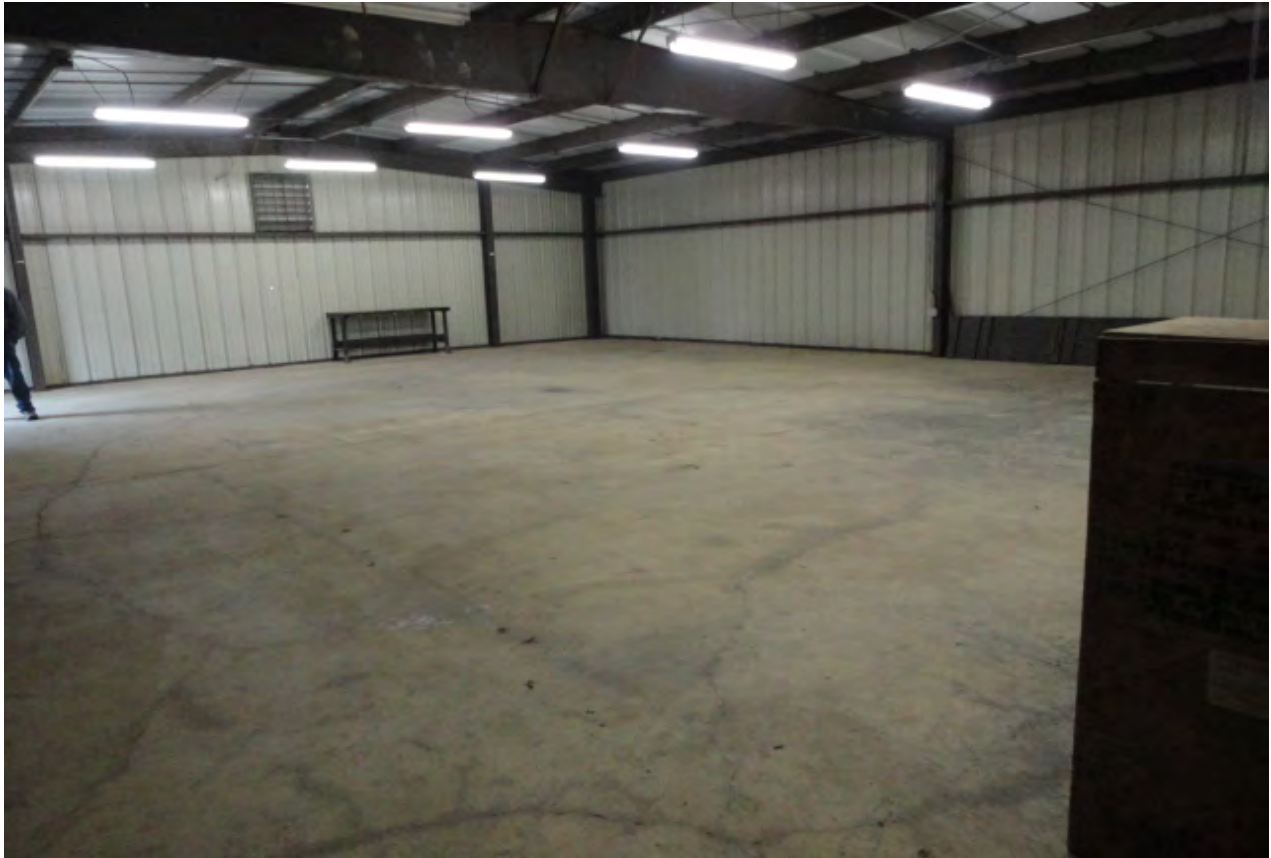
Photograph 25: View of the mostly empty interior of the large unit storage building.
