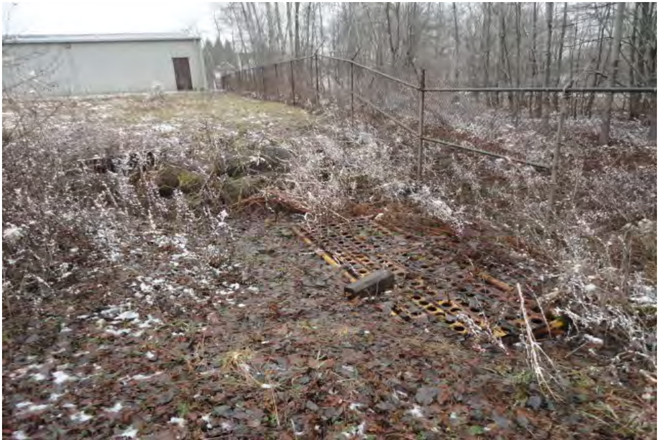
Photograph 30: View to the east of a stormwater drainage area along the southern fenceline. The former grease rack was reportedly located between this feature and the large unit storage building in the background.
