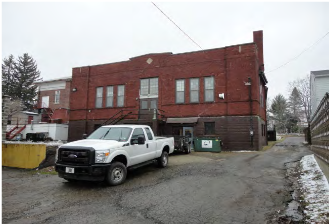
Photograph 2: View to the north-northwest of the rear of the RC building, paved driveway, and parking area.
