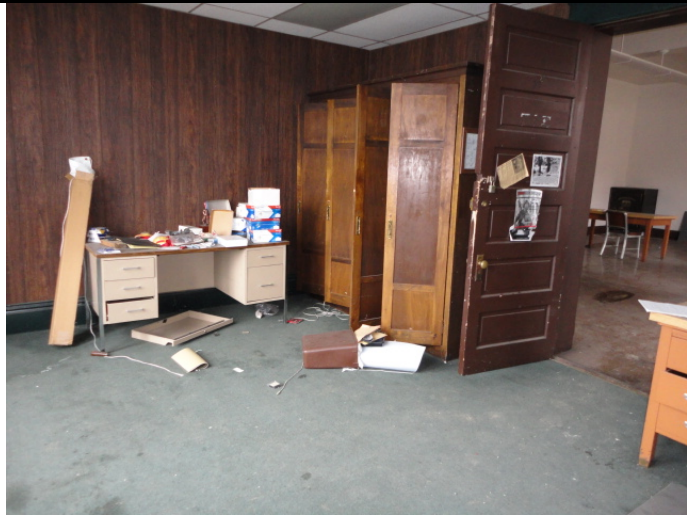
Photo 1 Front Offices, First Floor
